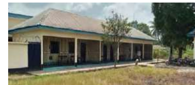
Ubeta CDF Project: Renovated Corpers Lodge
