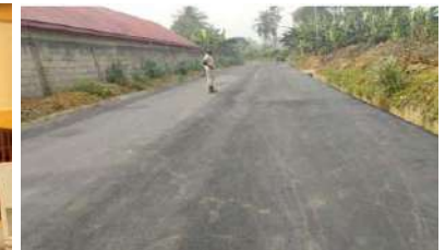
Rumuji CDF Project: 1Km Road
